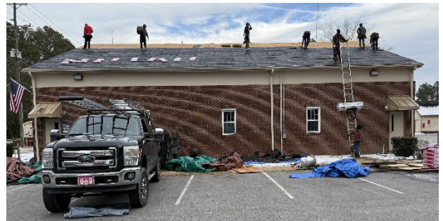
Apparatus Bay preparation and replacement of new shingles
