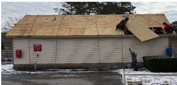
Storage Building preparation and replacement of new shingles
