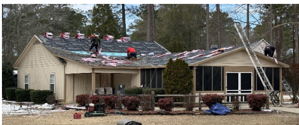
Picnic and Gym Facility preparation and replacement of new shingles
