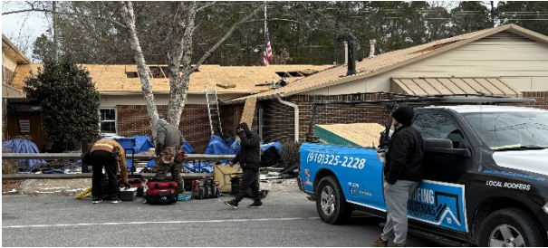
Administrative Roof preparation and replacement of new shingles
