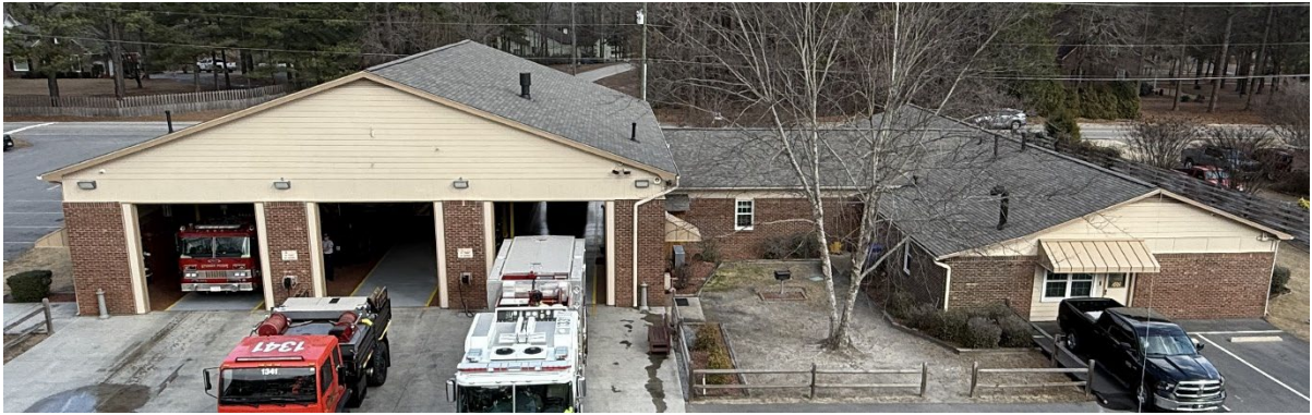
Station 13 New Shingles and Roof Main Complex
